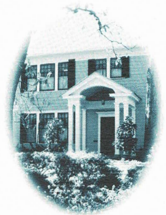
Theo S. Painter House Colonial Revival 105 West 32nd Street
