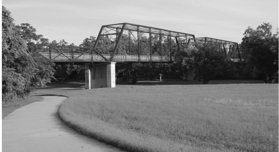
Moore's Crossing Bridge
