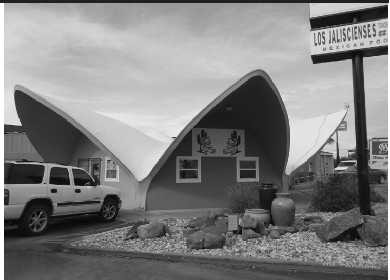
Taqueria Los Jaliscienses on US 290 East at Sheridan Avenue has a lotus-blossom roof, one of the more innovative and futuristic rooflines in Austin. The original windows for this Mid-Century Modern commercial buildings has had its windows replaced recently.
