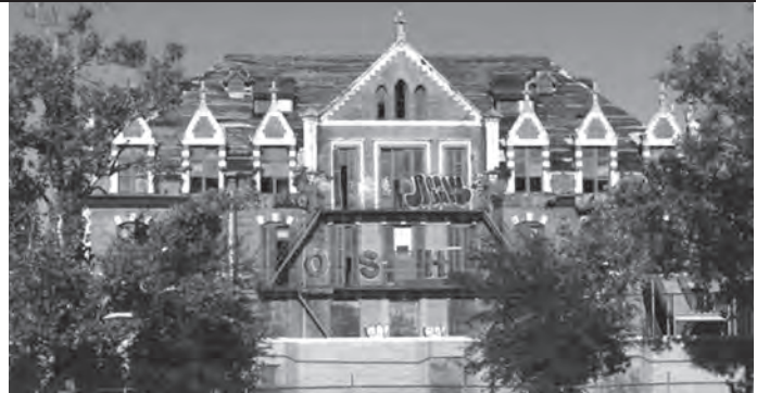
New Orleans' historic Bell School, part of an upcoming $36 million Artspace project providing affordable live/work housing for artists, cultural workers and their families ( artspace.org ).
