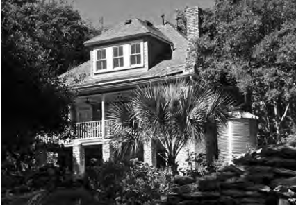
Splitrock's east façade overlooking Shoal Creek with solar array and rainwater & HVAC condensate collection tank (Photo BY Spec-All Products, Inc.)
