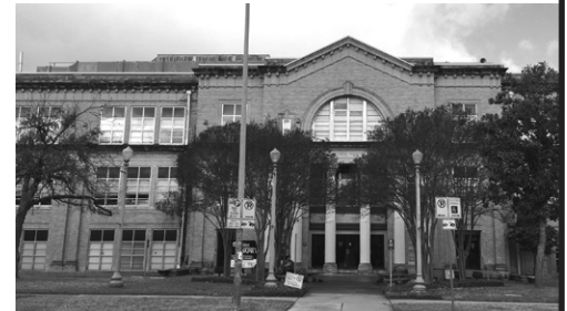
The former Austin High School
