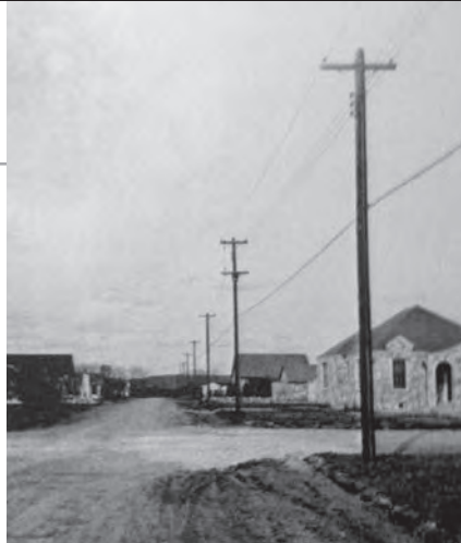
1937 Rosedale: Community infrastructure being installed.
