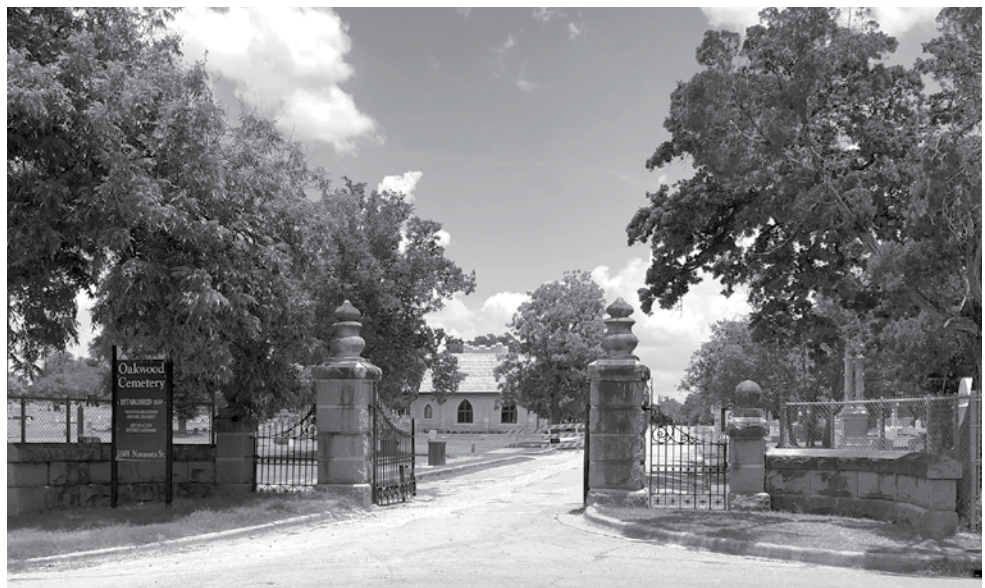
Oakwood Cemetery Main Gate (1908) before restoration.
