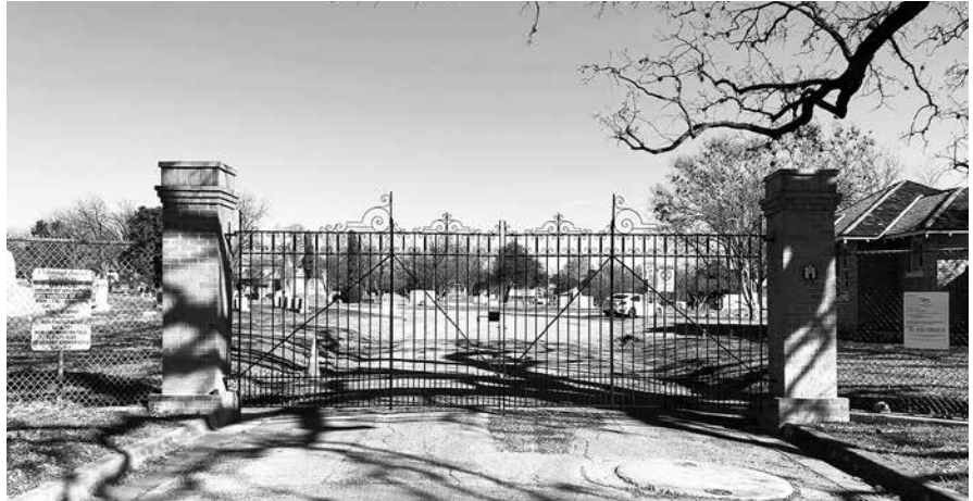
Oakwood Cemetery Annex's Main Gate (1916) after restoration.
