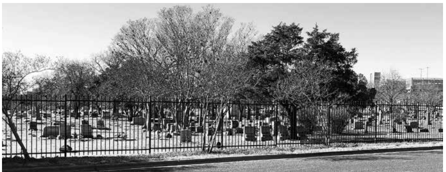
New steel fence to replace chain link and barbed wire.
