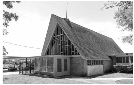
Prince of Peace Lutheran Church, demolished last fall.
