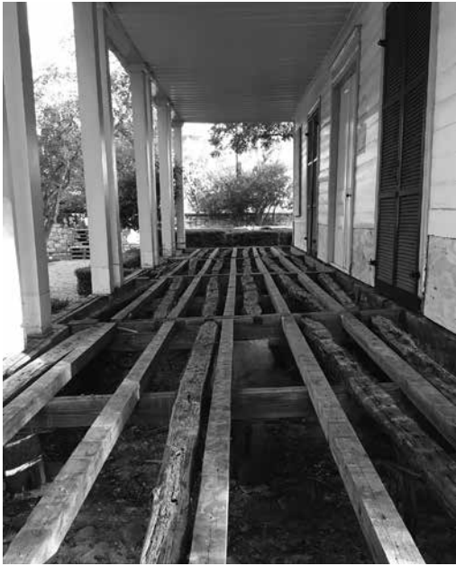
Cypress beams from the original 1841 construction lay beside newer materials.
