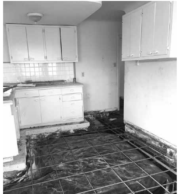
Kitchen before pouring the new slab.
