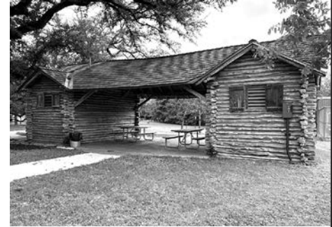
Shipe Park Shelter House
