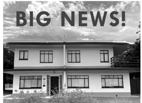
PA begins significant rehabilitation work on the McFarland House.
